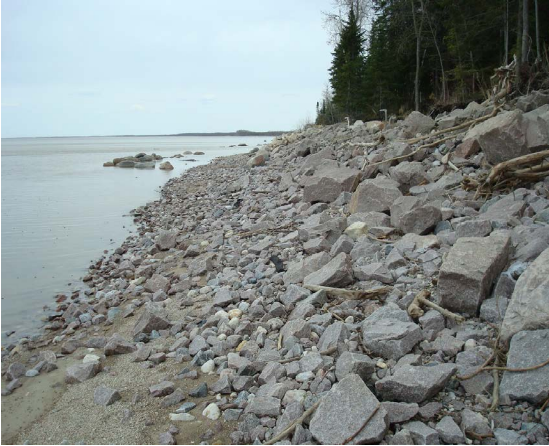
Stones washed out and slid down the bank into the water (photo taken by complainant)
